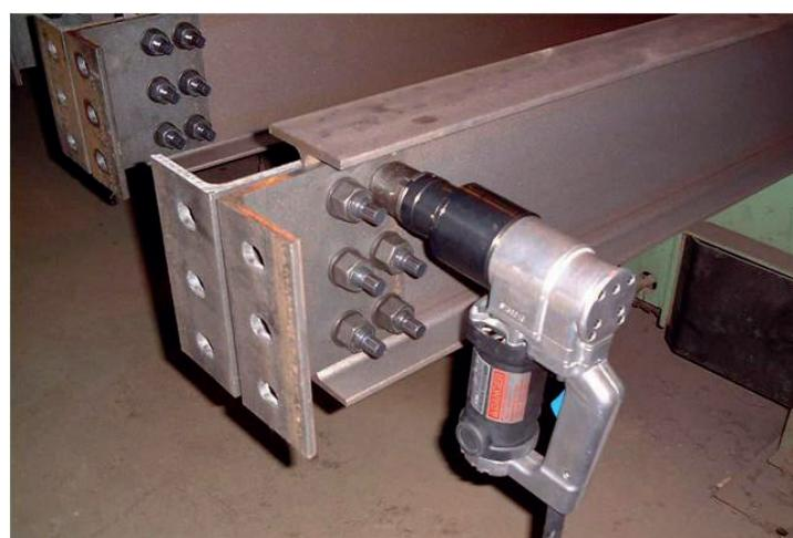
Calibration or adjustment of the wrench is not necessary, as the geometric and torque characteristics of the bolt automatically produce the required preloading into the joint.
